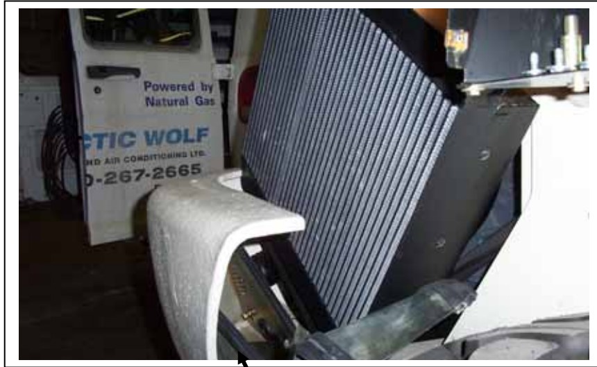
Bottom and front air dam unbolted and pulled away
